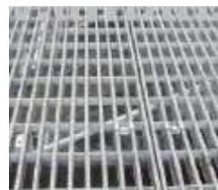
Grated Metal Decks
